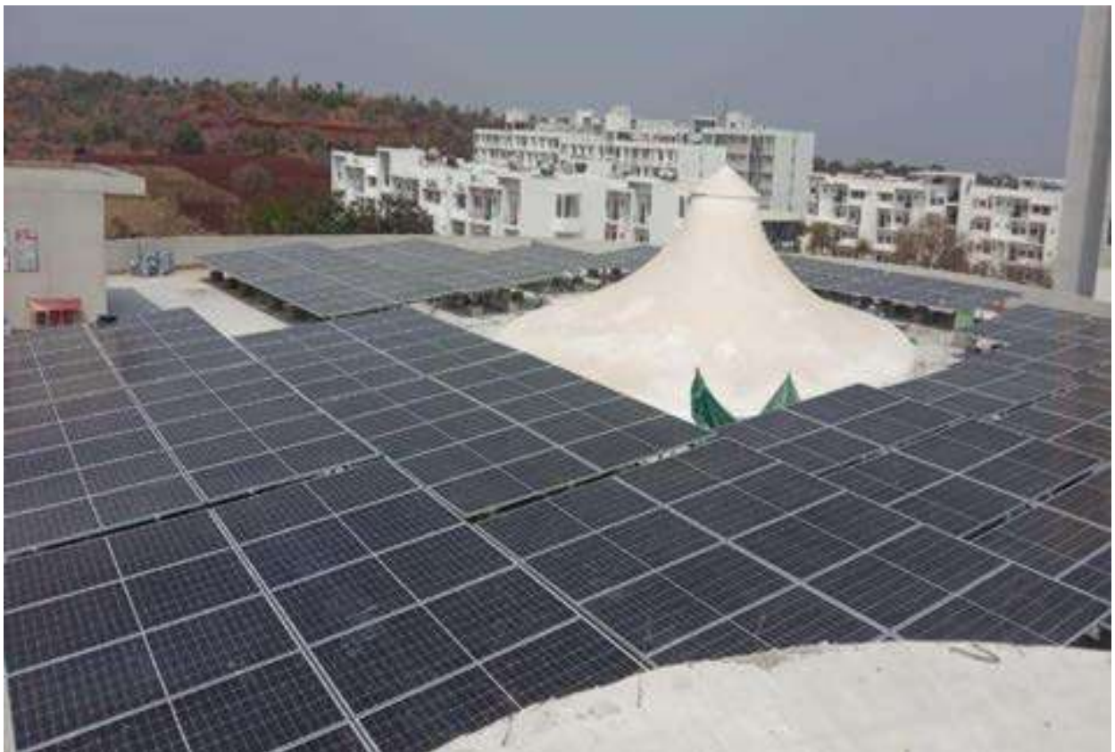
420 kWp Solar Setup (Phase -2)
